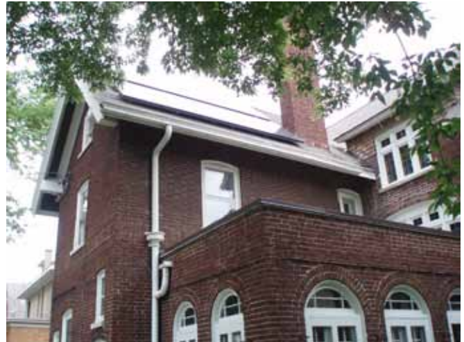
A solar panel system was installed on the rear elevation of this historic property in the Heritage Hill Historic District of Grand Rapids, Michigan. By locating the system in the rear of the property, the views from the public right-of-way remain preserved. (Image courtesy of Kimberly Kooles, N.C. Solar Center.)
